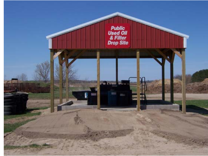
Wadena Station Located at the County Transfer Station 10542 170th Street
